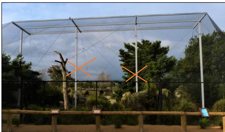
Figure 15 Avoid a structure with inside poles as support: Such inside poles can cause deadly collisions.
