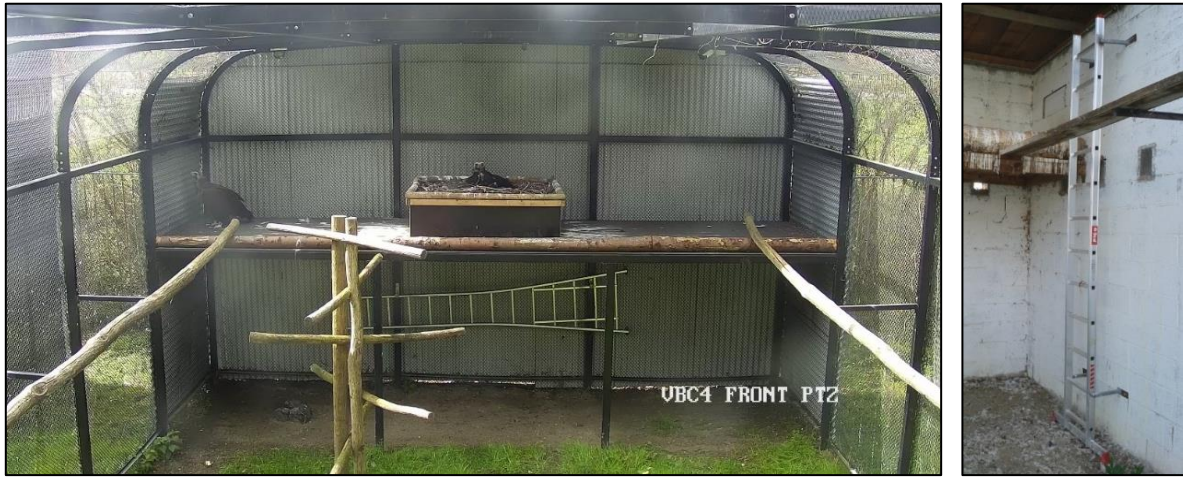
Figure 24 The ladder is fixed permanently under the nesting platform. When building a new aviary, it is important to foresee a good place to fix a ladder. This picture from the Bearded vulture husbandry guidelines shows a ladder fixed permanently in the aviary to the side, without having to move it.
