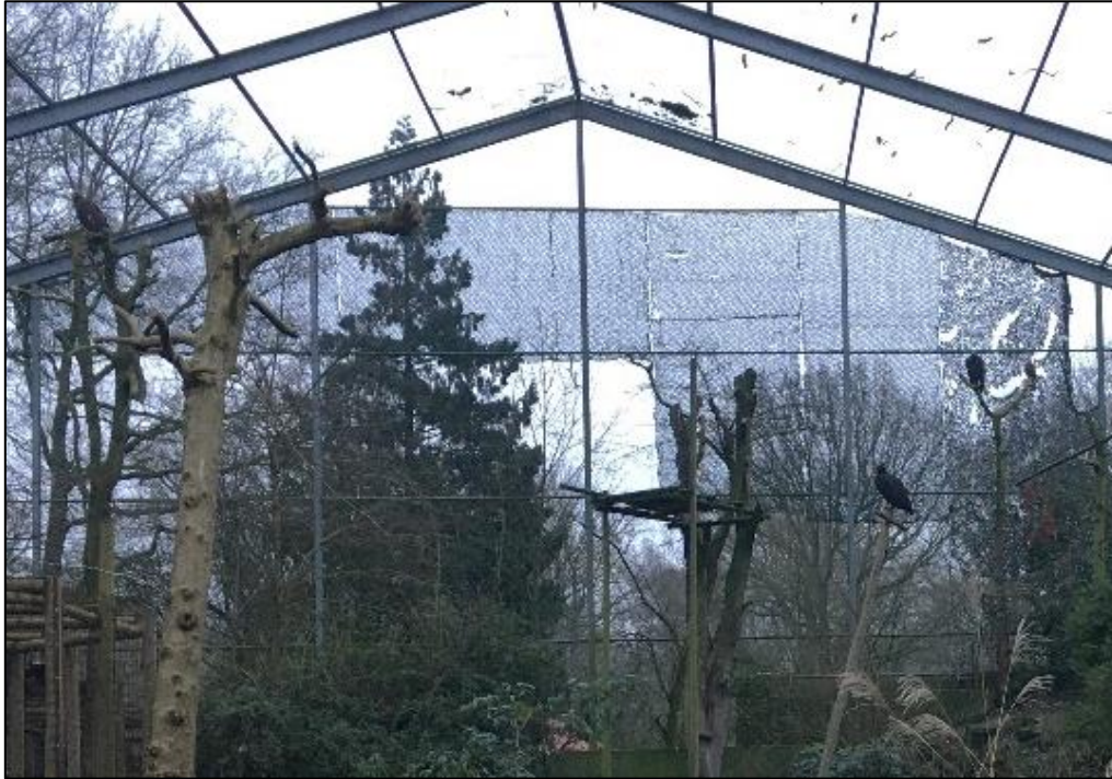
Figure 17 The inside area of the aviary is kept open in the socialisation aviary in Rhenen zoo and the fence is made more visible by using camouflage net, fixed at the outside of the aviary.
