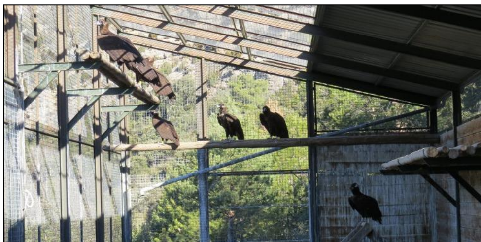
Figure 25 Boumort release aviary, Spain (Designed by Ing. Oriol Armet).
