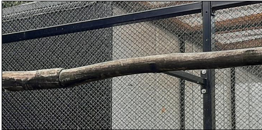
Figure 22 Perches are round shaped and have an average diameter of 12-14cm; they are mounted around the whole aviary.
