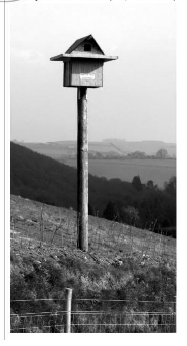
waterproof so the roof sheets should also be treated with Creosote or some other water-resistant preservative. The apex should be covered with a strip of aluminium or copper. The front, back and sides <u>MUST</u> overhang the floor of the box and as an extra precaution a large drainage hole (20mm - 3/4" - diameter) should be drilled in each corner of the floor of the box.
